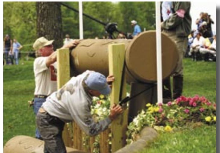
The broken styrofoam log on course was replaced in mere minutes.
